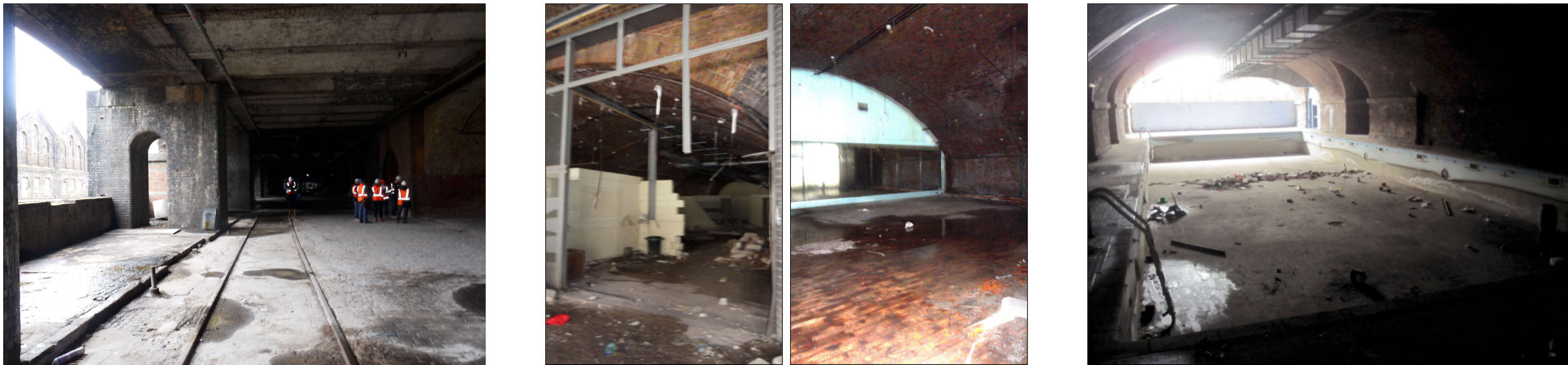
EXAMPLES OF VARIATION IN FLOOR LEVEL AND FINISH - Existing condition to be addressed to enable all units to have level access off London Road.
